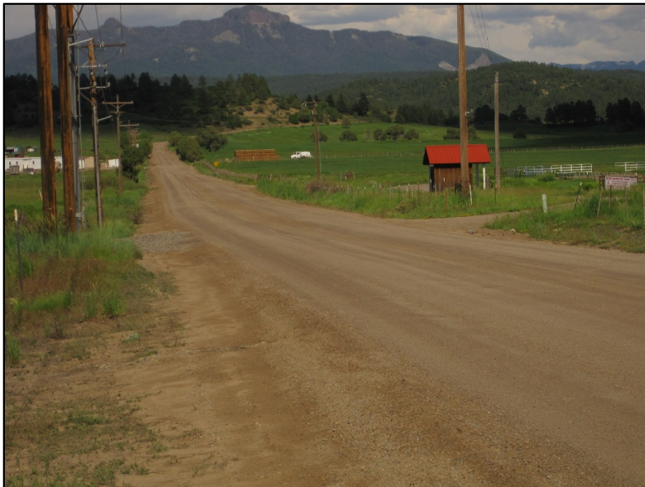
Photo 2. Portion of Mill Creek Road survey area looking east from near the intersection with Highway 84 (2015)
